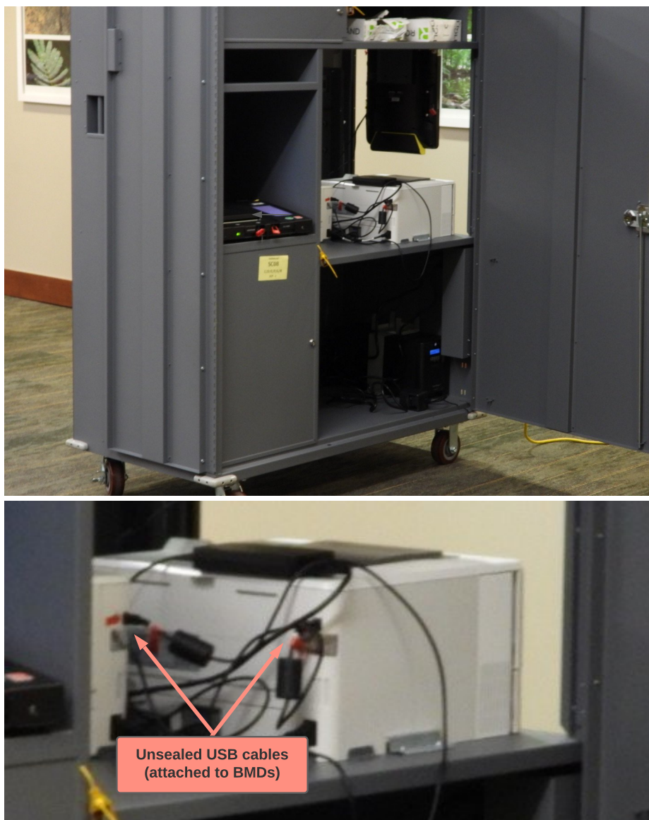
Figure 9: ICX USB Interfaces are Exposed to Voters and Unsealed. A USB cable connects the BMD to an off-the-shelf laser printer. At polling places, the end of the cable attached to the printer is physically accessible to voters, and it is not protected by a tamper-evident seal. Voters could install malware on the ICX by attaching a device to the end of this cable. Photograph taken by Harri Hursti during polling place observation in Fulton County, November 3, 2020.
